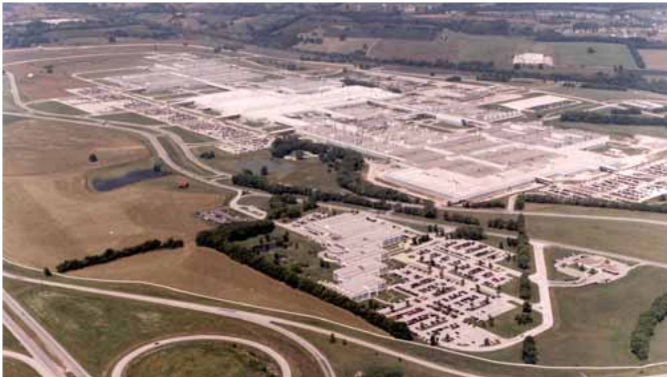
The GM assembly and manufacturing plant
