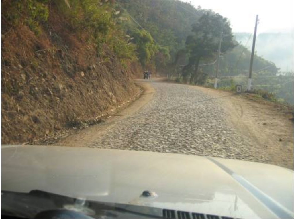
Photo 3: Secondary road (hand-laid rock surface) in rural Gengma County, Yunnan Province
